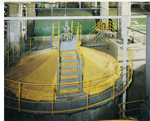
Wastewater treatment facility
